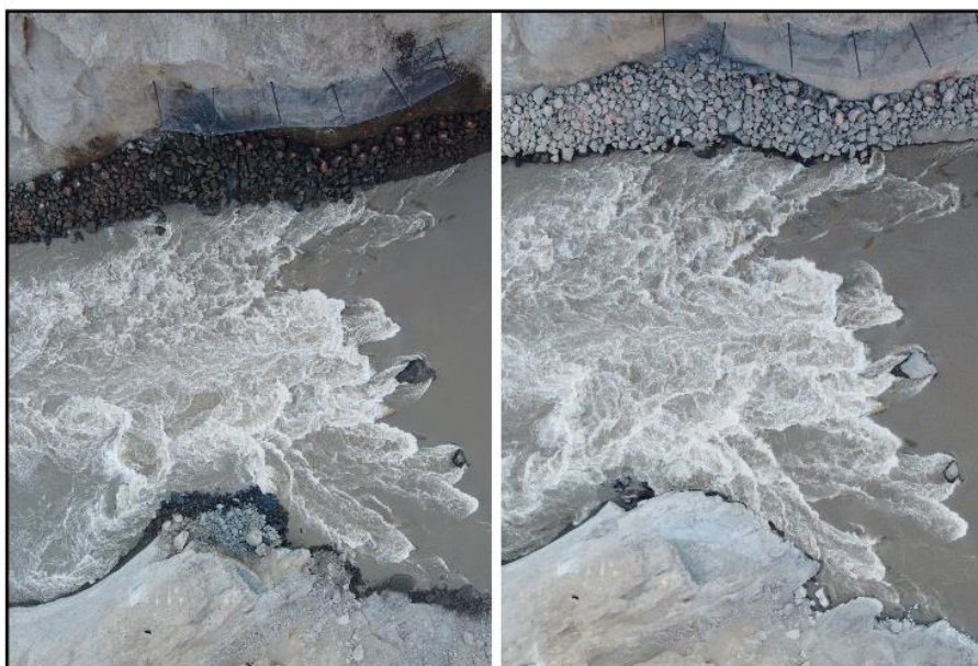
PICTURED: (L-R) A comparison of the East Toe before and after blasting that occurred on April 11, 2020. At higher flows, the river will be widened significantly.
