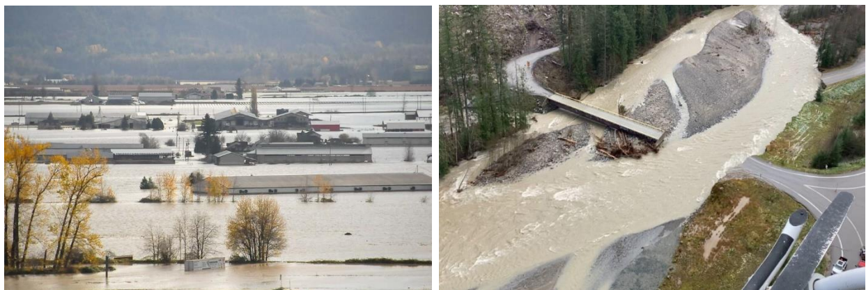
November 2021 Flood Devastation in Southern British Columbia
